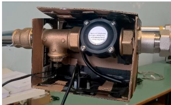
Fig. 4 - Representation of Box A installed.
