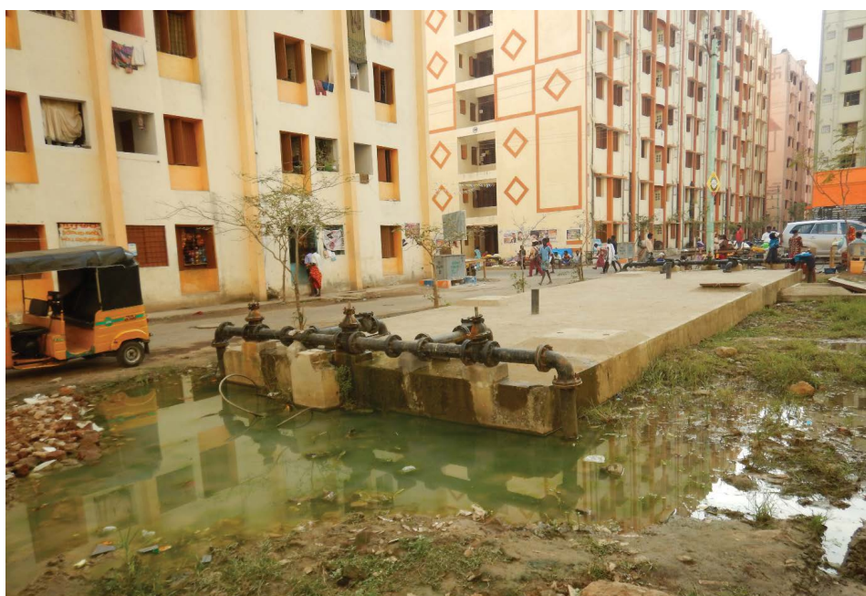
Figure 2: Housing built on marshy land is usually water-clogged which could have health implications in the long term
