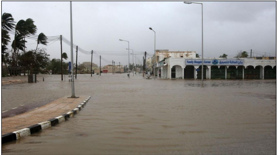
Figure 19. Flash floods and damages during Cyclone Mekunu 2018 (Alwatan, 2018)
