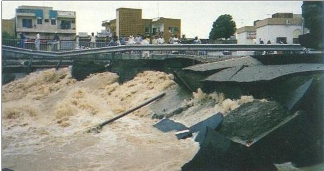
Figure 16. The impact of flash flooding on one of the roads during Cyclone Gonu. NCSI, (2015)
