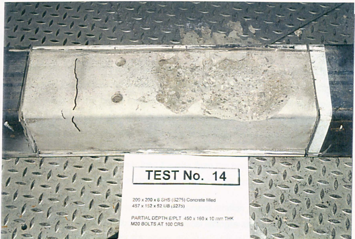
Figure 6.4 Steel tube cut away to reveal concrete spoiling and cracking for test number 14
