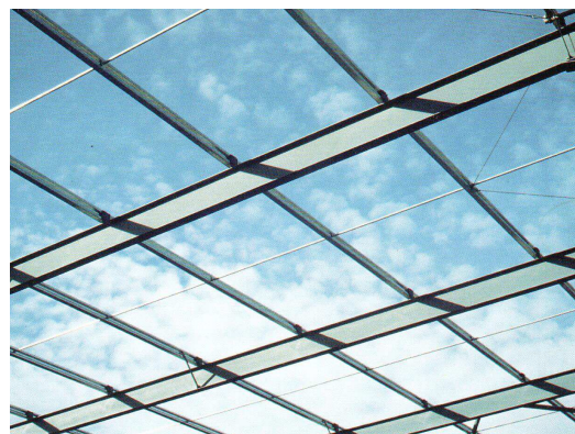
(b) Purlins supporting roof sheeting
