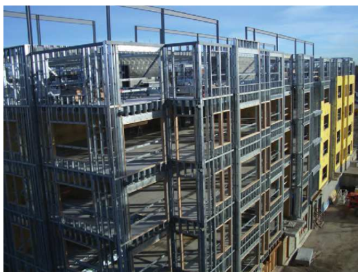
(a) Light steel framing
