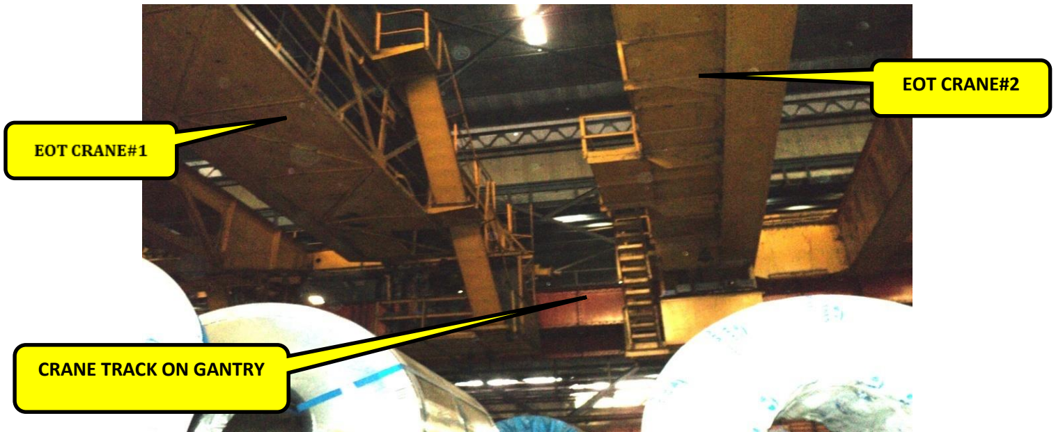
Fig 5.8. Two Working Eots Working Very Close On Same Gantry
