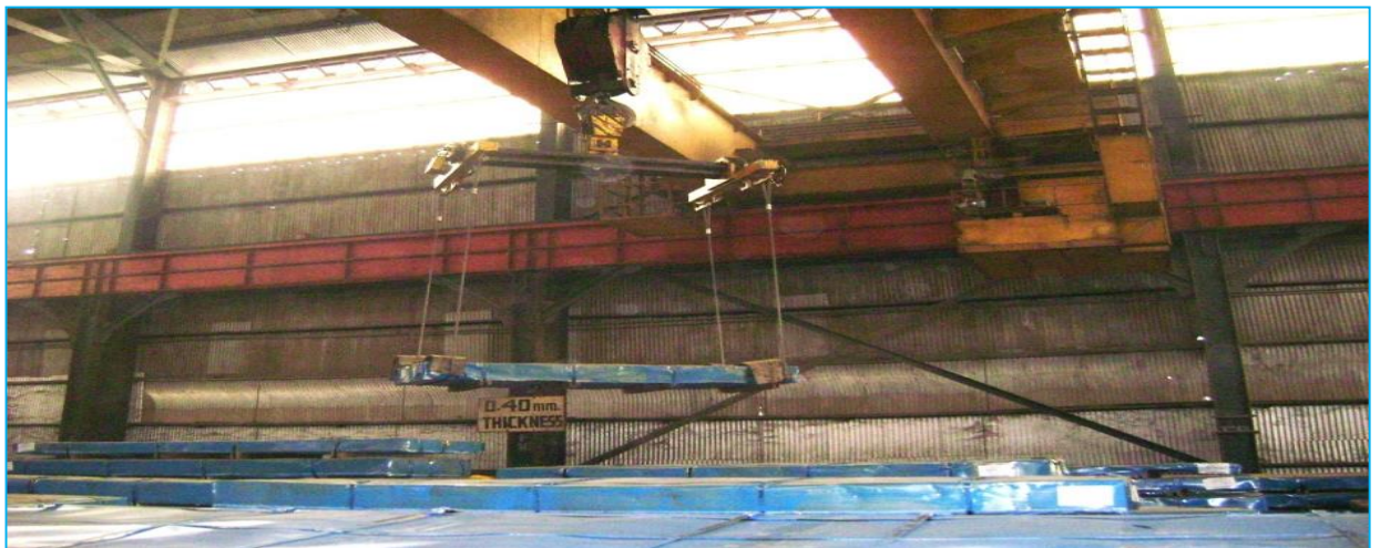
Fig 1.2. MATERIAL HANDLING WITH EOT CRANE USING SLINGS
