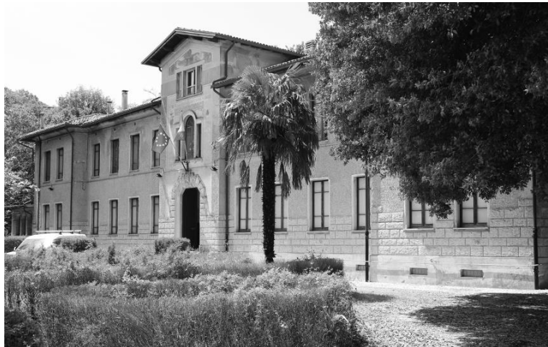
Figure 36: Photograph of the historical building (Cercato and De Donno, 2018).
