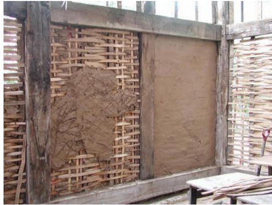
Figure 2.4: Walls of Wattle and Daub [6].
