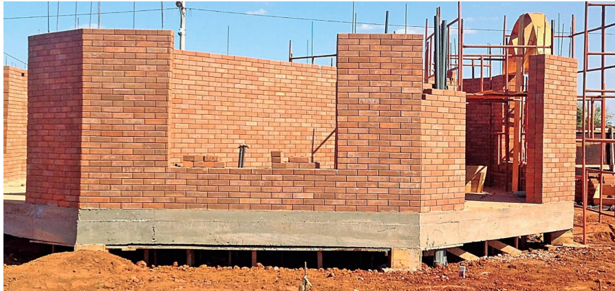
Figure 2.6: Construction of walls with CEB [17].
