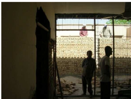
Fig. 18 Workers are demolishing some parts of an original PEH due to heterogeneity of local materials and those applied in original PEHs
