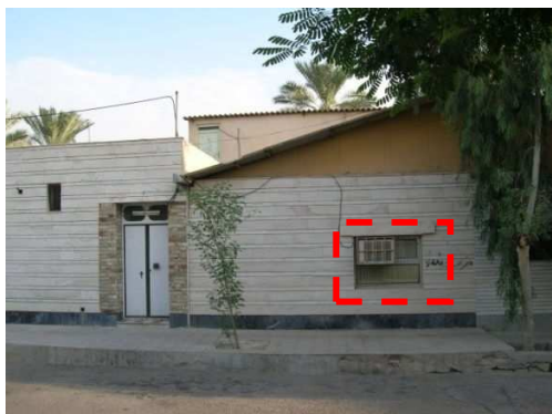
Fig. 14 An instance for the applied electrical active air-conditioning system in Lar
