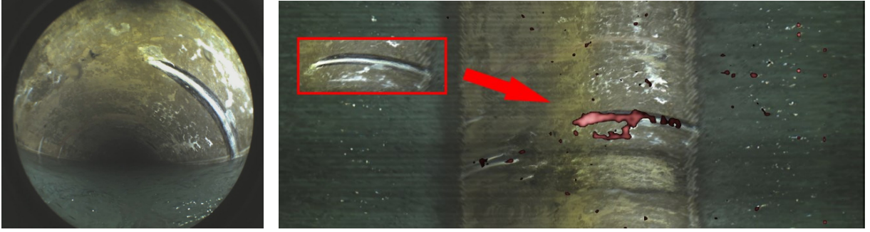
Fig. 13. Left: visual appearance of an anomalous leak, as seen from the camera. Right: unfolded view, with highlighted anomalous areas detected by the system. The actual leak, covered by the anomaly map, is shown in the red box.
