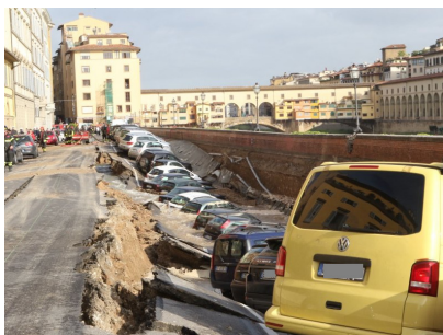
Fig. 1. A ground collapse due to a waterworks leakage.
