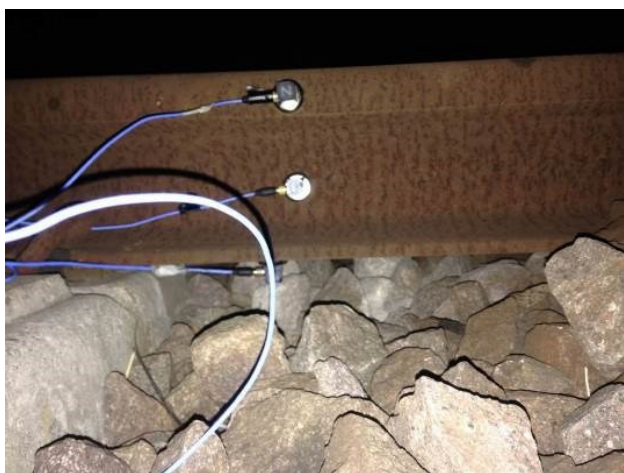
Figure 8: Real accelerometers installation.
