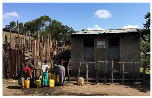
A water point was installed in 2012 as part of a biogas development initiative in an informal urban community of 200 households. The facility provides sanitation, gas for cooking, and organic fertiliser. It consists of four latrines and an inlet for animal waste, a fermentation chamber where the biogas (methane) is produced, and a communal kitchen with four stoves. The slurry byproduct is rendered safe by fermentation and used as fertiliser for the community garden.
