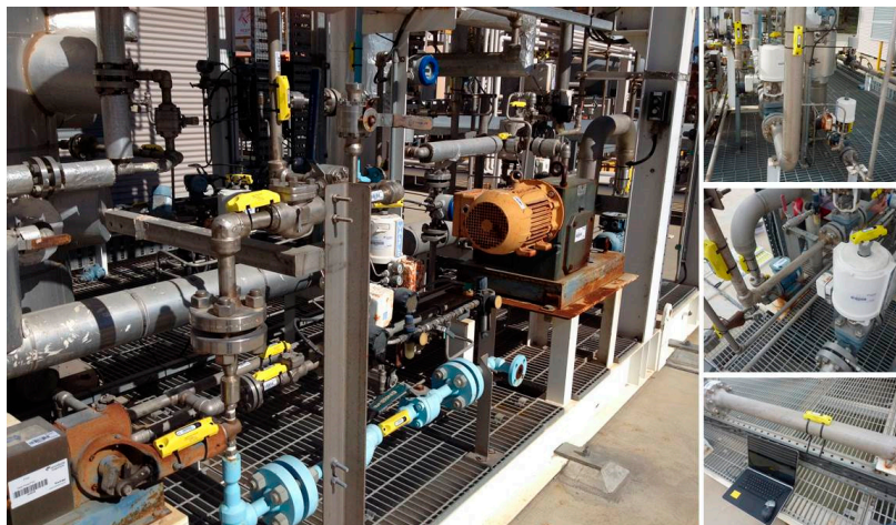
Figure 10. The attachment of RFID tags on the dehydration module.
