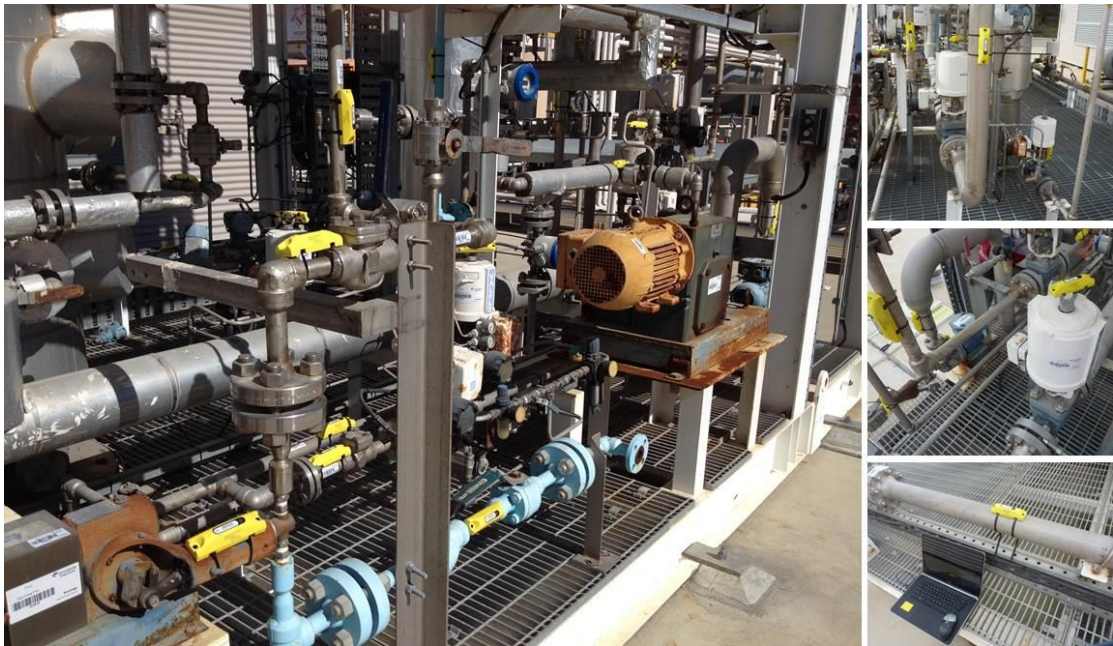
Figure 7-10: The Attachment of RFID Tags on the Dehydration Module
