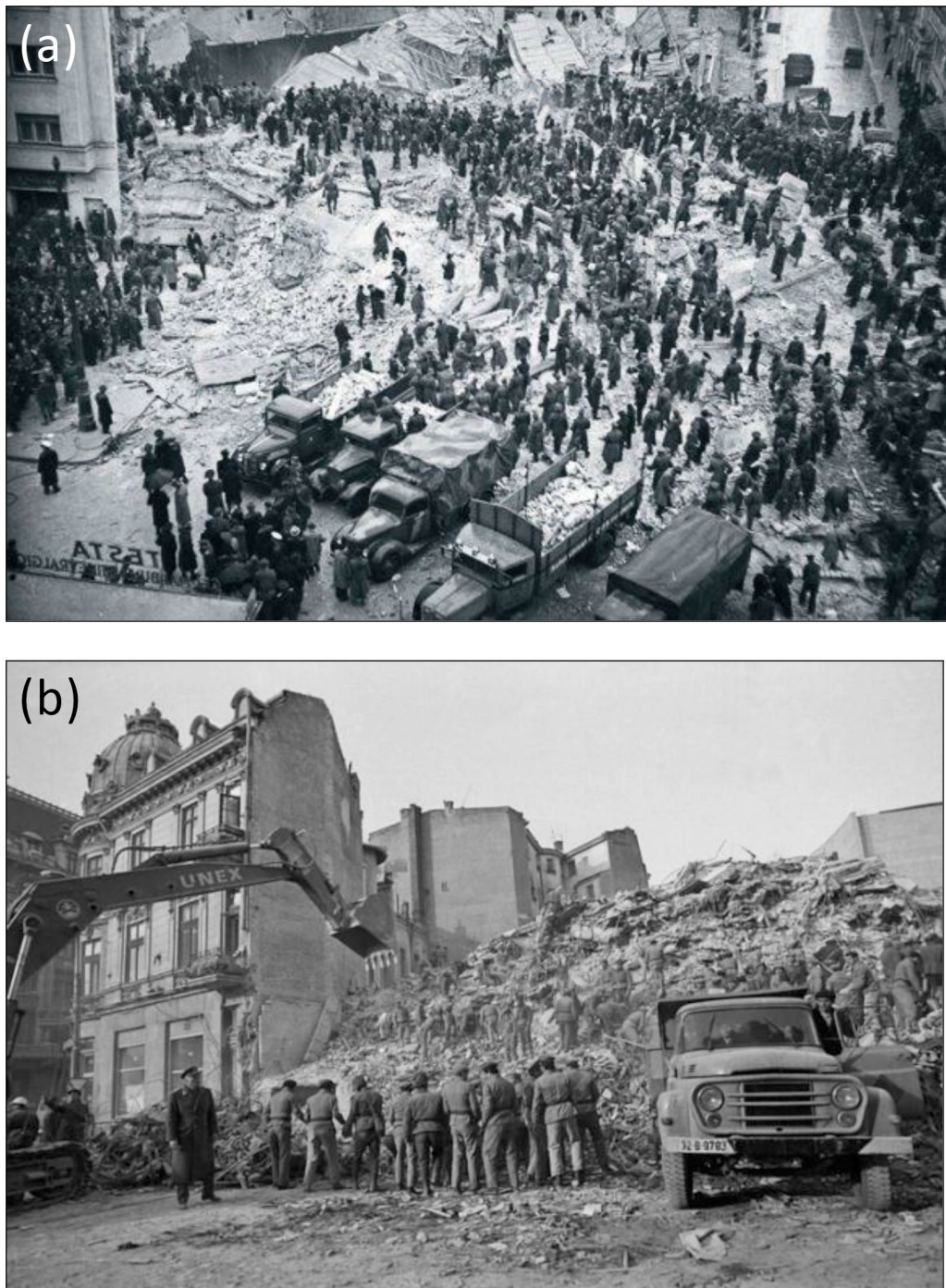
Figure 2. (a) The collapse of the Carlton block in Bucharest in 1940. Source: https://upload.wikimedia.org/wikipedia/commons/6/60/Iosif_Berman_-_Marele_cutremur_din_anul_1940.jpg (last access: 3 June 2017). (b) The collapse of the Continental block in Bucharest's historical centre in 1977 blocked the access streets, so clearance was delayed by more than 12 h. Source: Agerpres.
