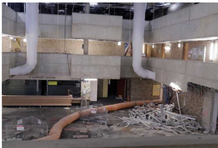
Fig. 11 An example of recycle material on-site sorted and stored
