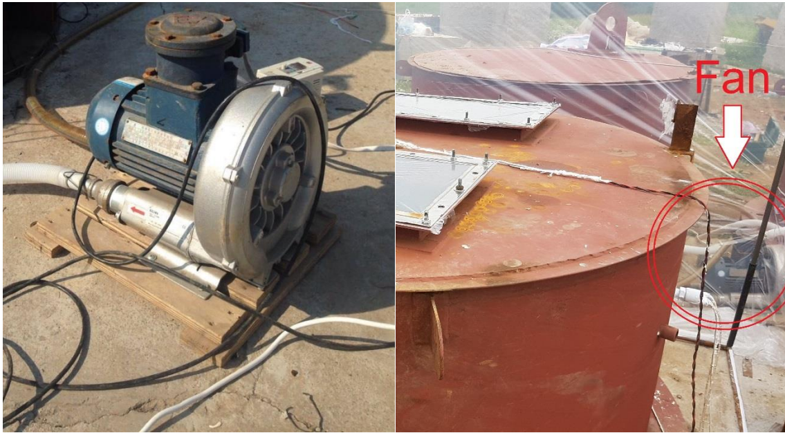
(a) Fan for gas mixing for the center tank
