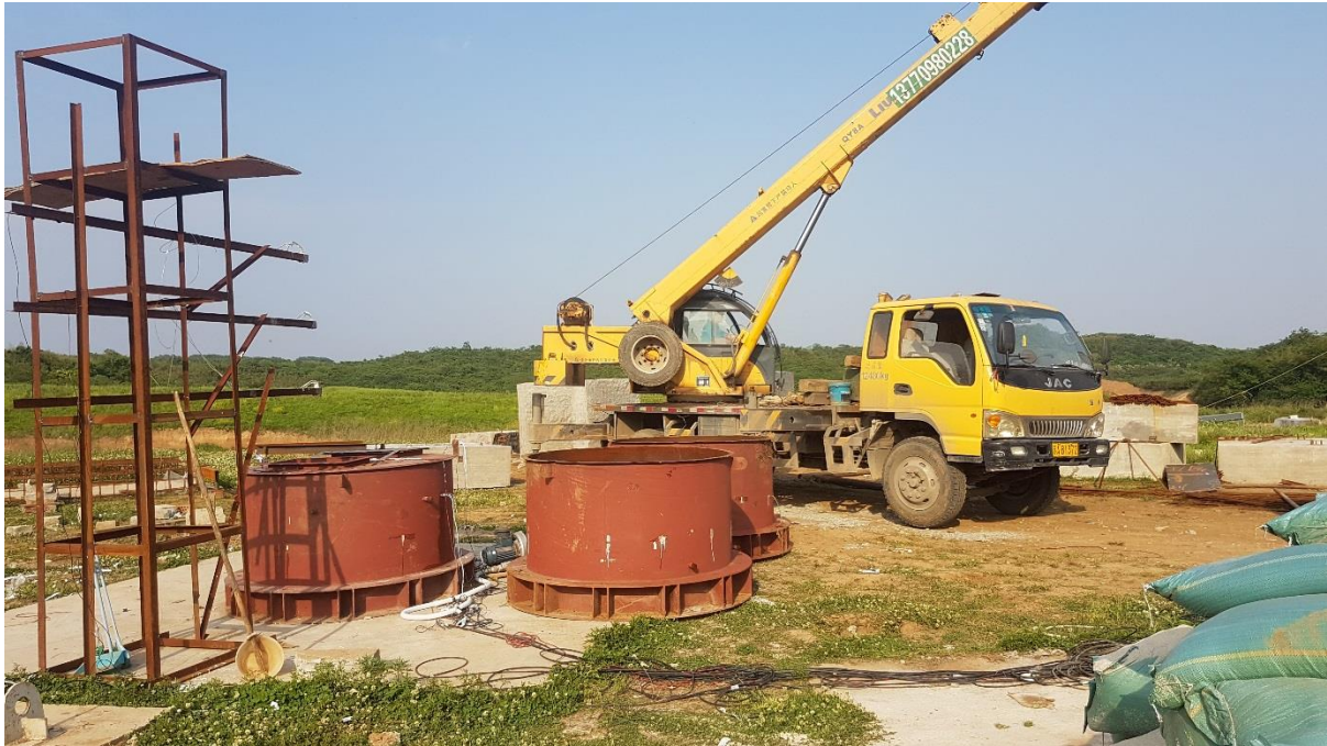
(a) Hauling of tanks by using a crane truck to arrange the tank group layout
