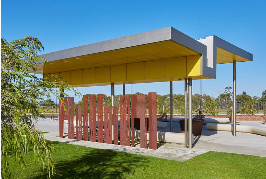
Figure 6-47. Forlano, Penelope. Marri Healing , Corten steel screen and soffit, photo by Douglas Mark Black, 2017.
