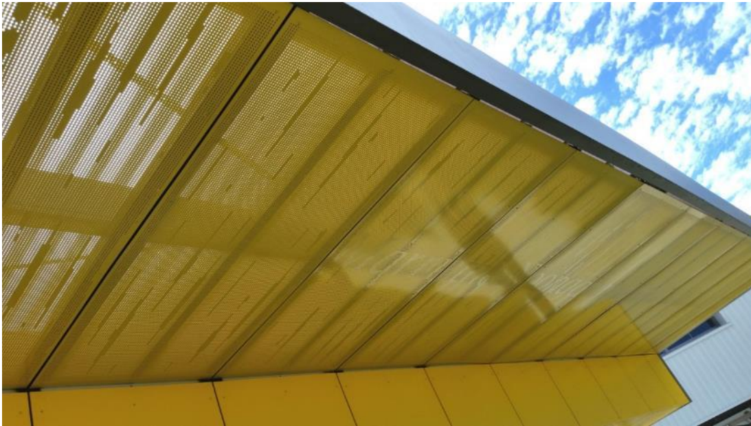
Figure 6-45. Forlano, Penelope. Marri Healing (soffit), 2017. Dimensions: 9,030mm W x 1,965mm D. Materials: 4mm thick powder coated aluminium.
