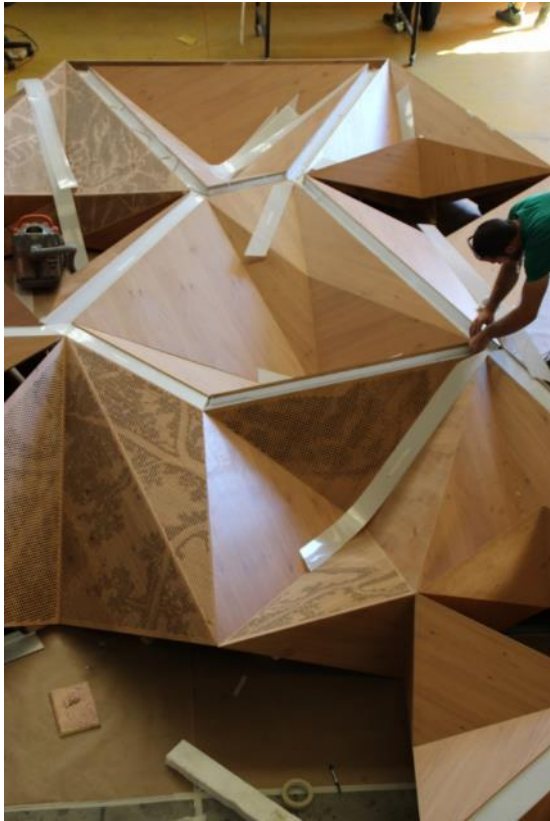
Figure I-14. Forlano, Penelope. Construction of artwork, 2014.
