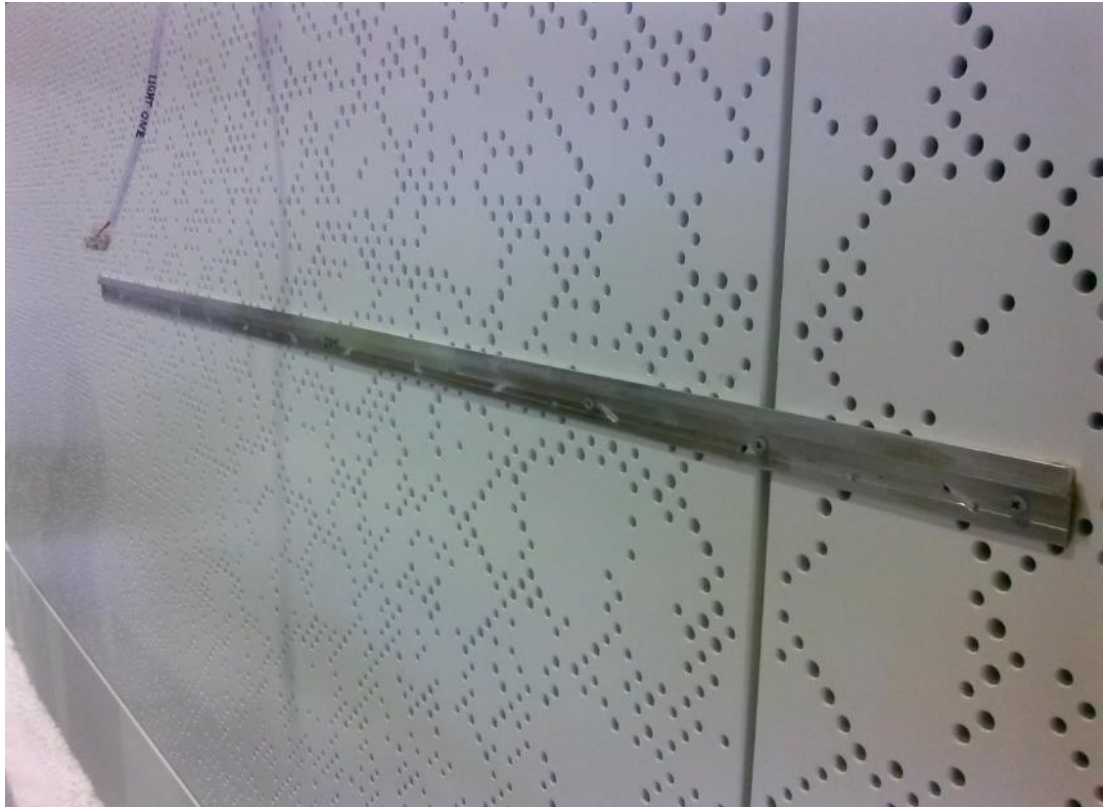
Figure I-17. Forlano, Penelope. Installation of artwork, detail of perforated wall and aluminium hanging system, 2014.
