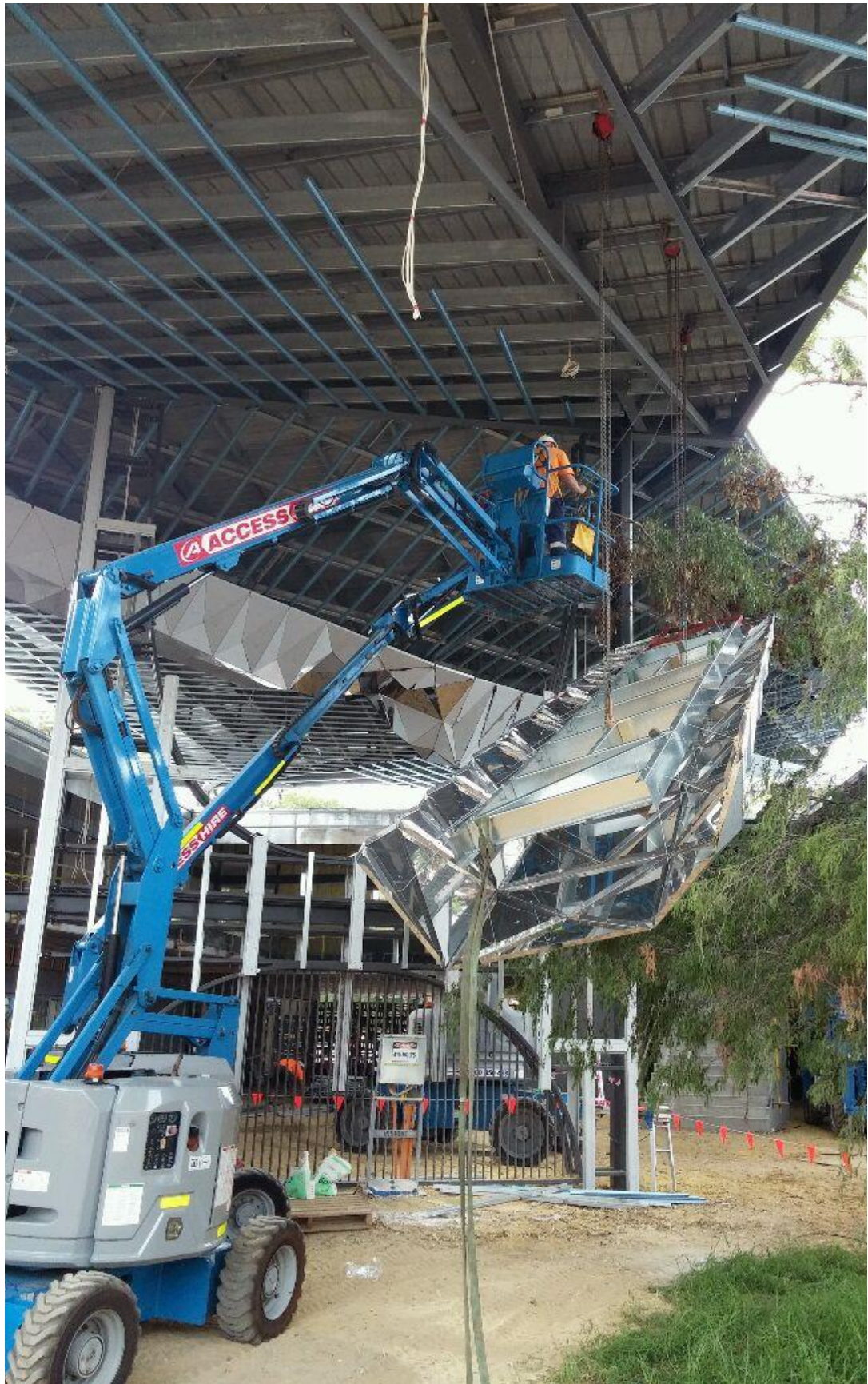
Figure I-41. Forlano, Penelope. Kaleidoscopic Wave , component F, being installed, 2017.
