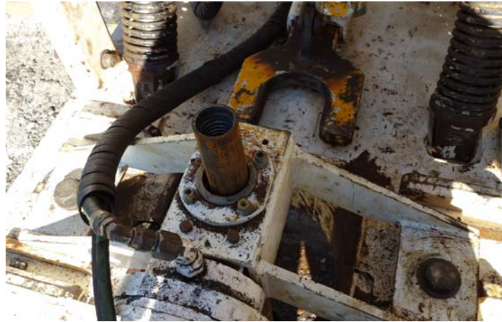
Figure 6.10 Disconnection of drill pipe to drop prepared cuttings.
