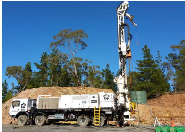
Figure 6.2 Drilling rig for the field tests.
