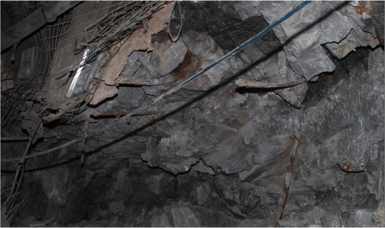
**Figure 19 – Reinforcement retention inconsistency due to poor resin encapsulation at the collar likely caused the first metre of rock mass instability to preferentially load the surface support.**
