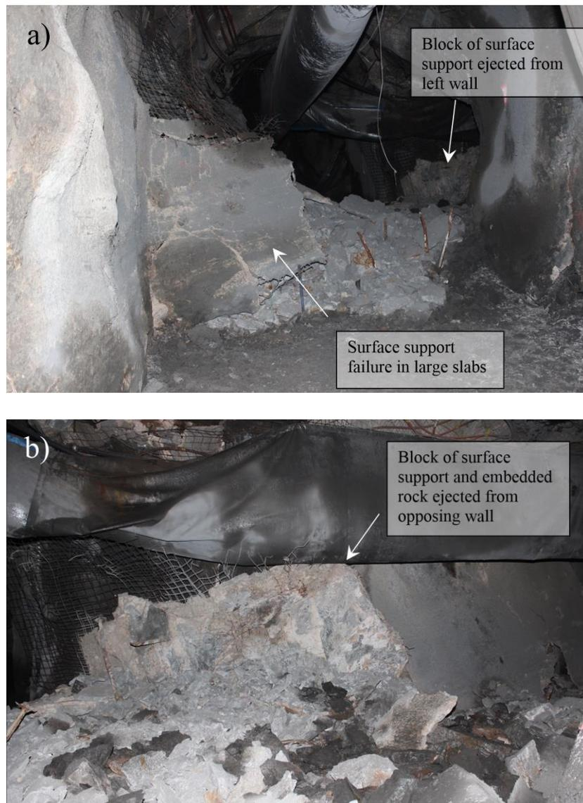
Figure 14 - Failure of ground support scheme leading to violent, very high velocity ejection.
