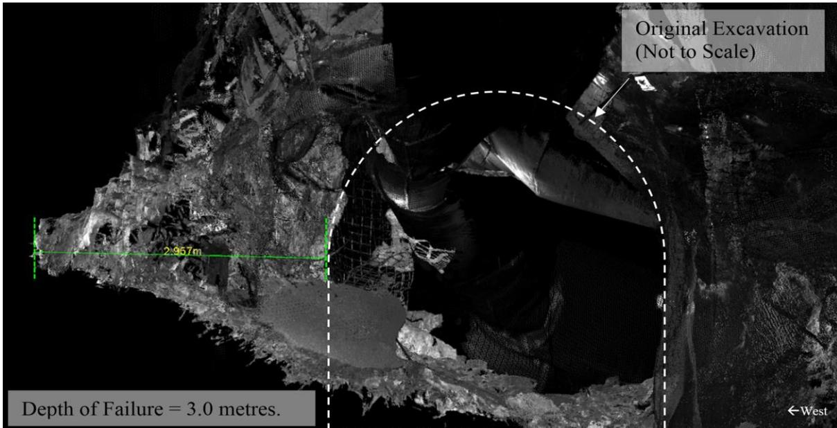
**Figure 18 - Maximum depth of rock mass failure of 3.0m caused by sudden violent event.**
