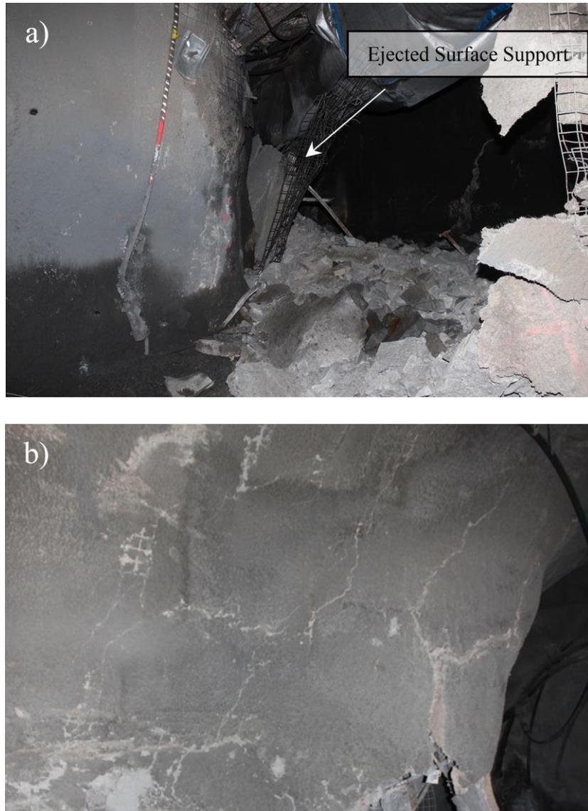
**Figure 15 - a) Surface support damage after extremely high loading demand, b) surface support damage after low to moderate loading demand. Fracture pattern reflects reinforcement spacing with bolt locations where cracks intersect.**
