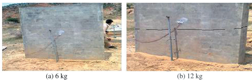
FIGURE 6. Blast loaded wall after explosion.
