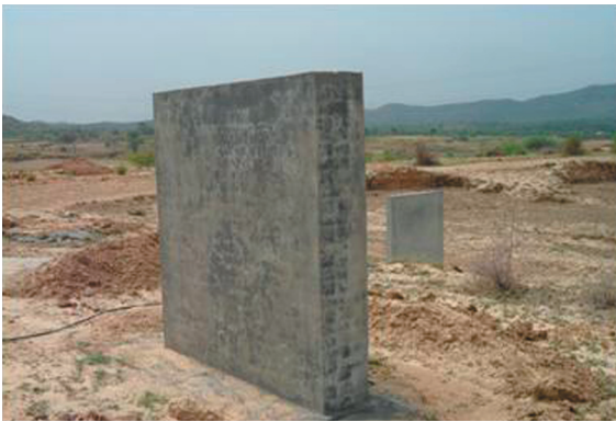
FIGURE 1. View of brick masonry wall.
