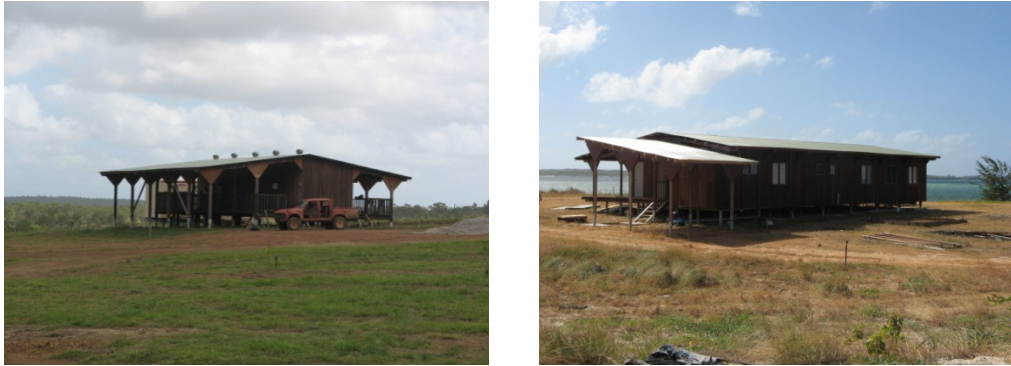
FIG. 2: BUNK HOUSE AT GARRATHIYA AND LIVING QUARTERS IN DHANAYA
