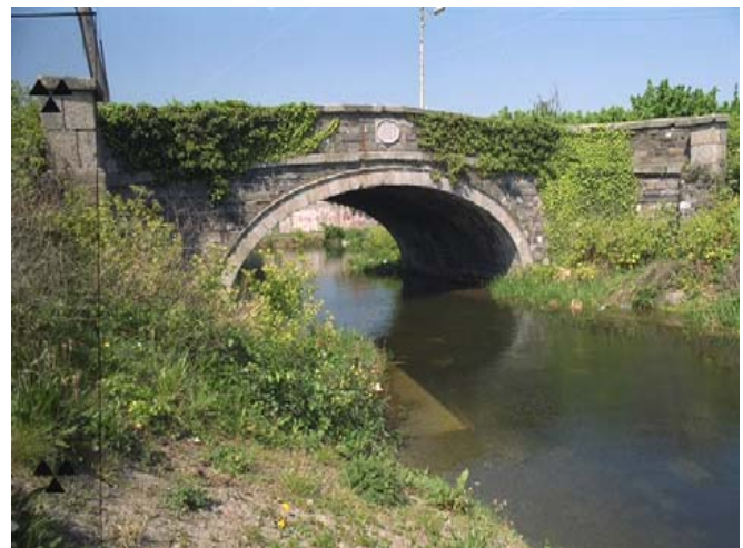
Fig. 1 Griffith Bridge – Dublin
