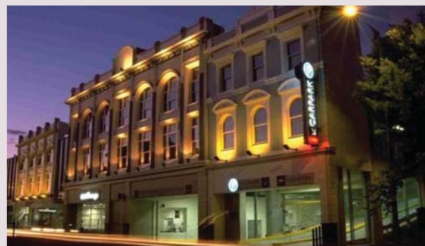
Figure F-11: Christchurch Bus Xchange, Lichfield Street
