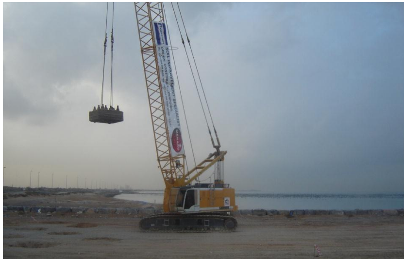
Figure 2. Application of dynamic compaction on Marjan Island
