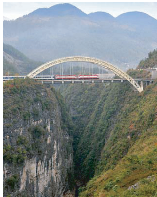
Figure 1. A photograph of the Yeshan River Bridge
