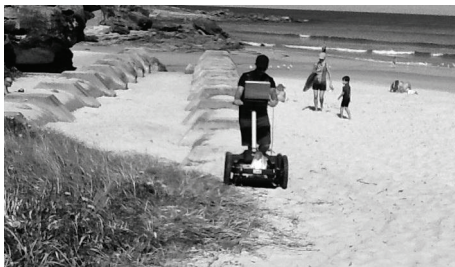
FIGURE 12: GPR along the concrete pipe at Freshwater Beach (profile P3).
