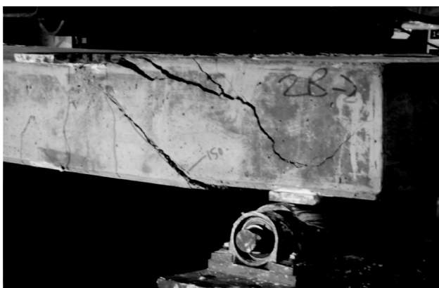
Figure 7. Spalling of the concrete above the top reinforcement
