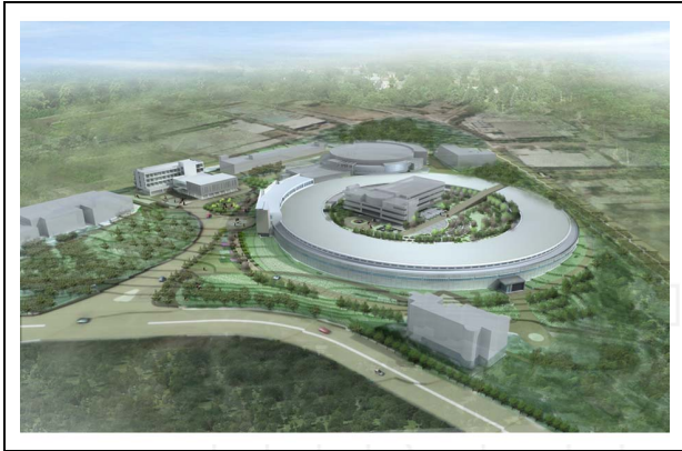
Figure 12. The as-built overall view of TPC [20]
