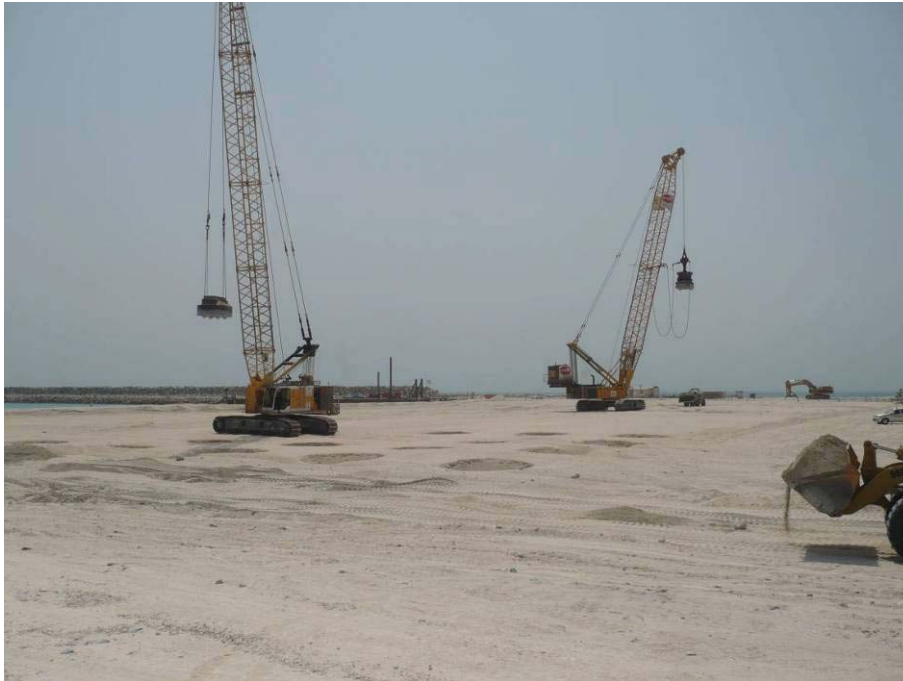
Figure 2. Dynamic Compaction using 28 ton and 35 ton pounders
