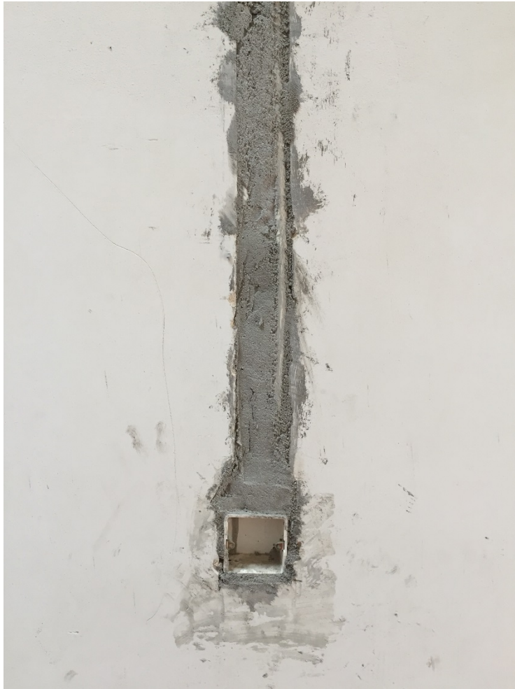
Figure 8. Electrical services are not integrated into the 3-D printing process by WinSun.
