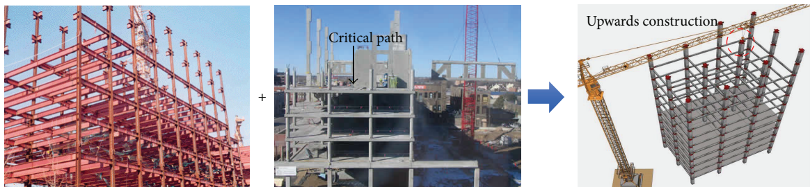
FIGURE 5: Reduction of the hybrid precast frame construction period.
