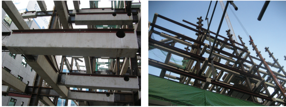
FIGURE 1: Building construction with hybrid precast frames.
