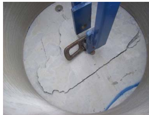
(b) View into liner showing lifting clutch
