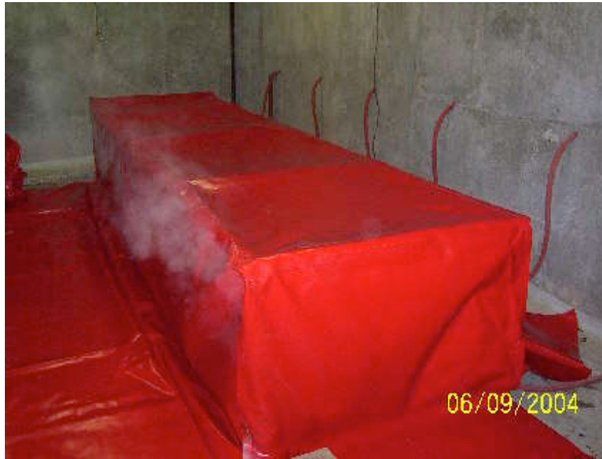
Figure 3.15: Steam Curing in Progress
