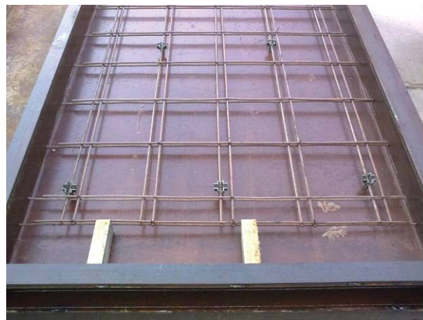
(b) Reinforcement in Formwork
