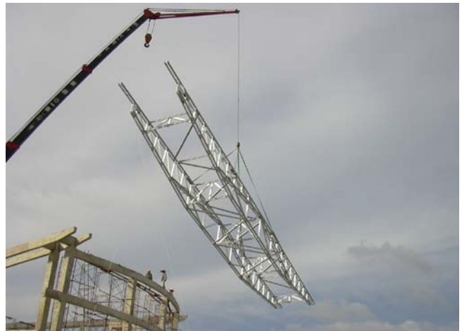
Figure 6: Lifting of truss
