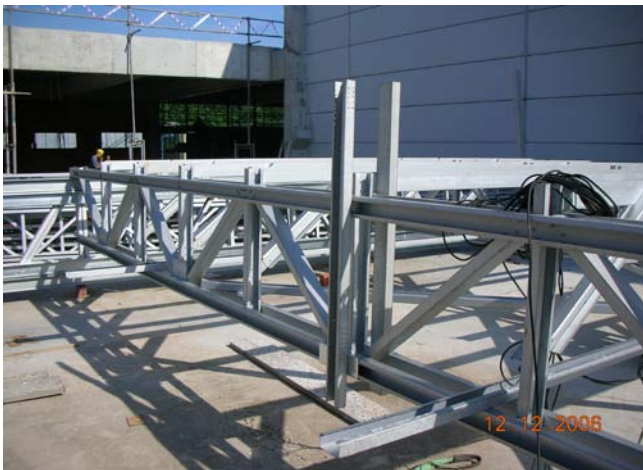
Figure 5: Top and bottom chords built-up sections
