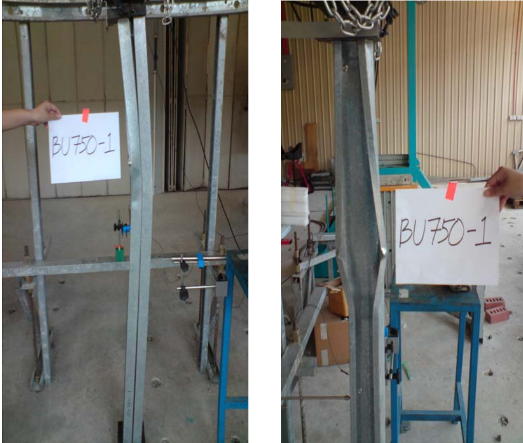
Figure 8: Buckling mode of column
