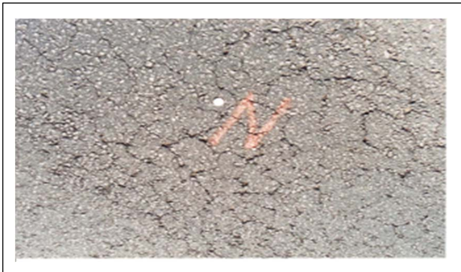
Figure 2.3 – Fatigue Cracking
