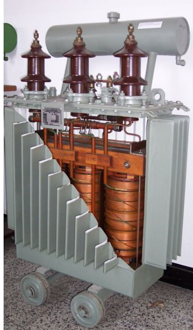
Figure 2-1: Three-phase oil-cooled transformer with cover cut away.
