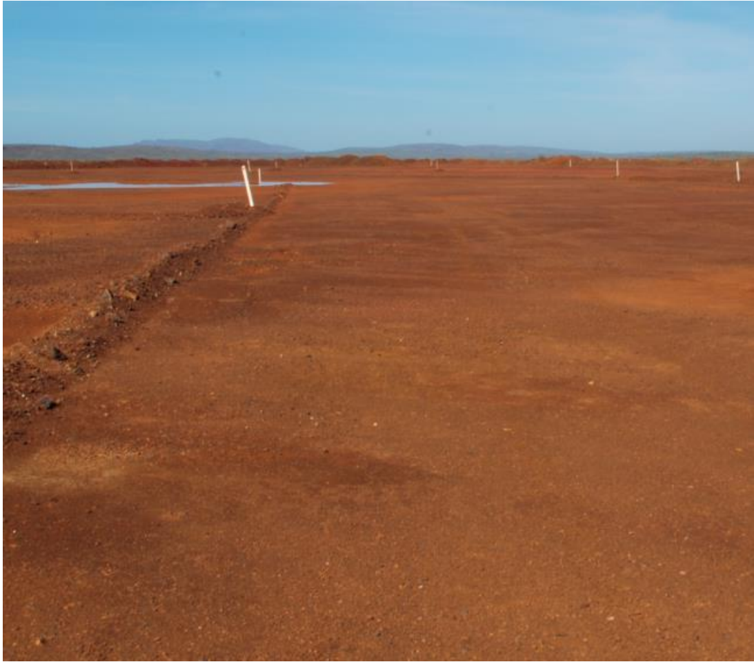
Figure 3.10: Section 1, looking from chainage 80m back to zero.
