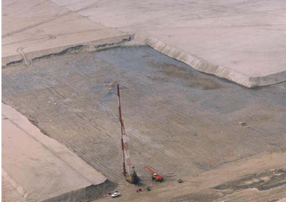
Figure 5.7 Aerial view of surcharge close to vertical drain installation works.
