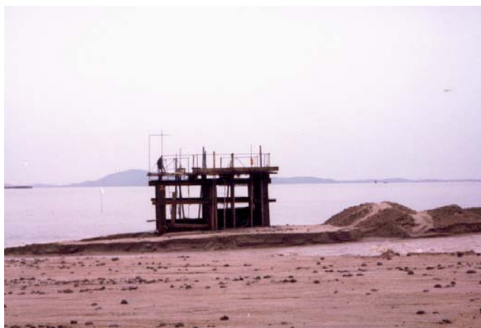
Step 6: Reclamation proceeding towards protection platform
