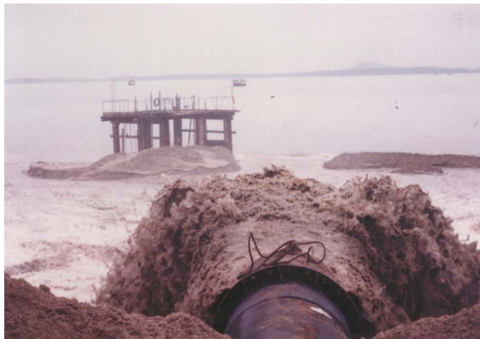
Step 5: Sand pumping towards instrument platform
