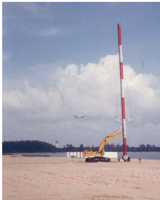
Figure 5.4 Vertical drains installation works at project site
