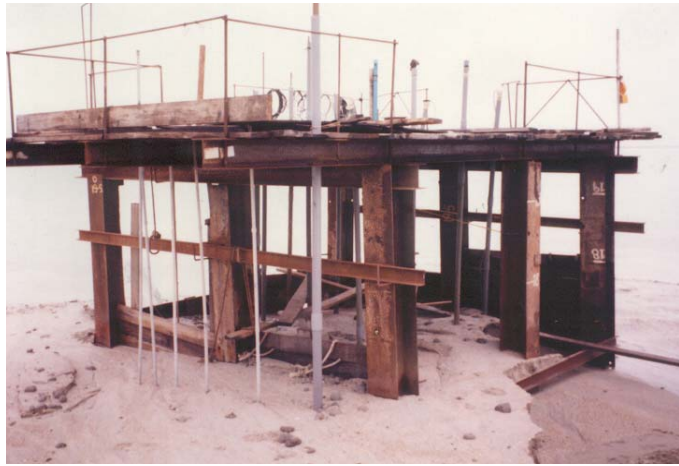
Step 7: Filling to platform level
