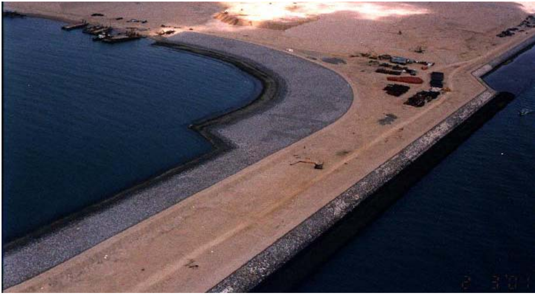
Figure 4.9 Aerial view of shore protection works.
