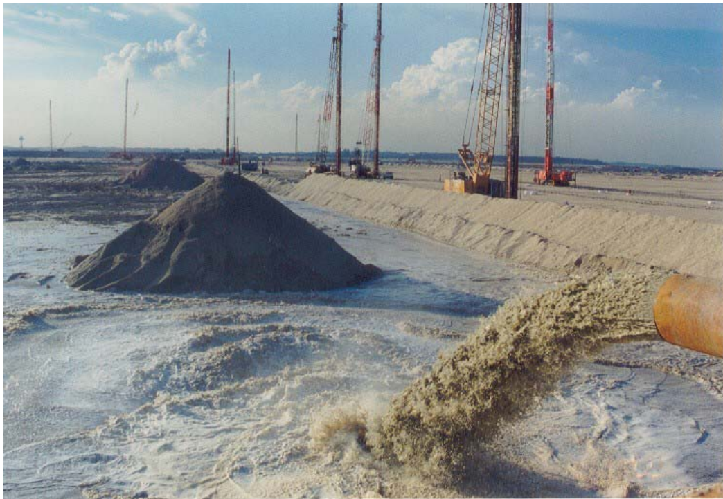
Figure 4.3 Land reclamation sand-pumping operations.
