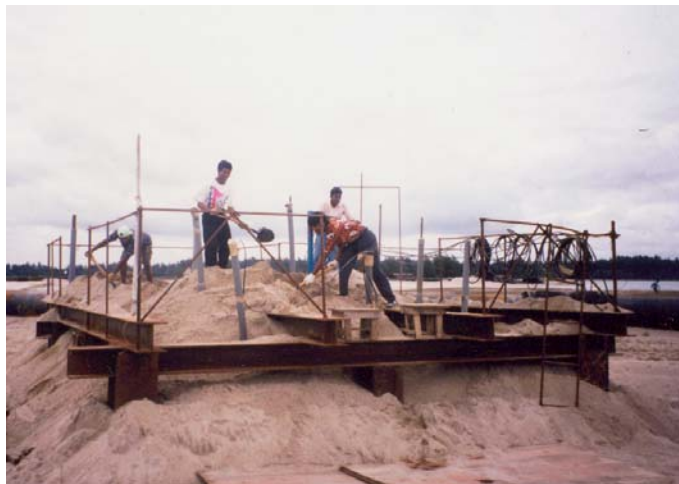
Step 8: Preparation for final surcharge fill
