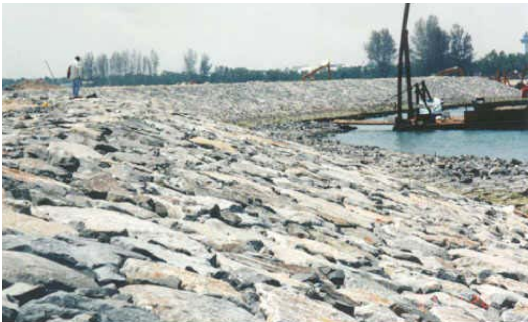
Figure 4.10 Close-up view of shore protection works.
