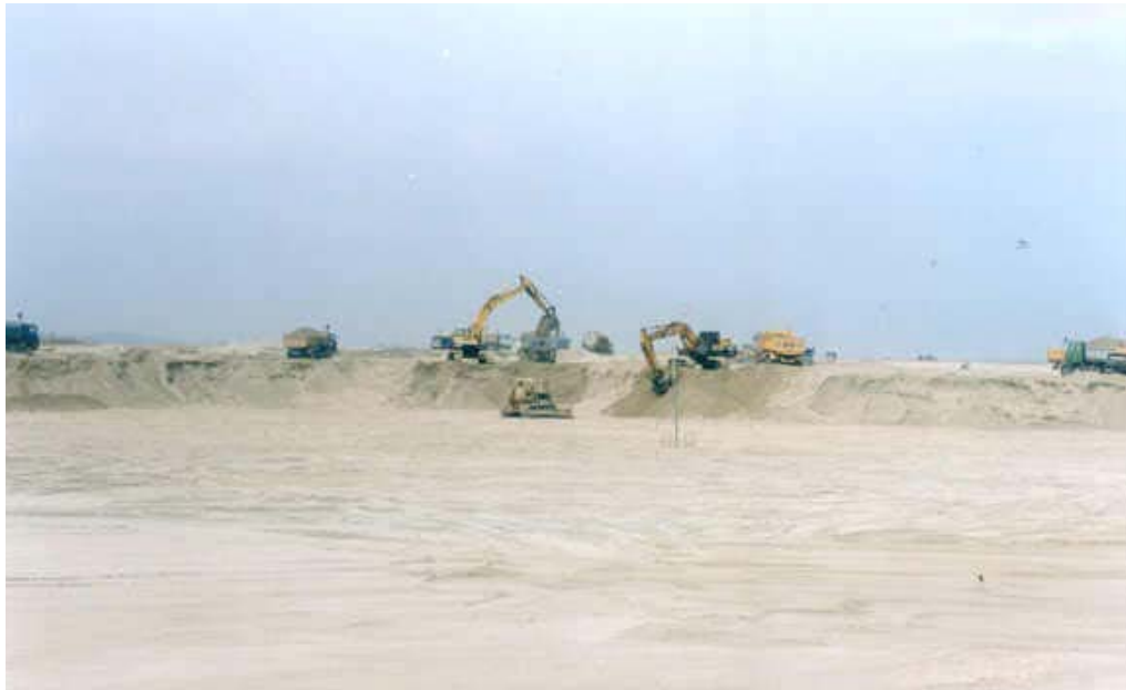
Figure 5.6 Surcharge placement operations at the project site.
