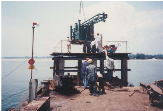
Step 4: Boring-rig for instrumentation
