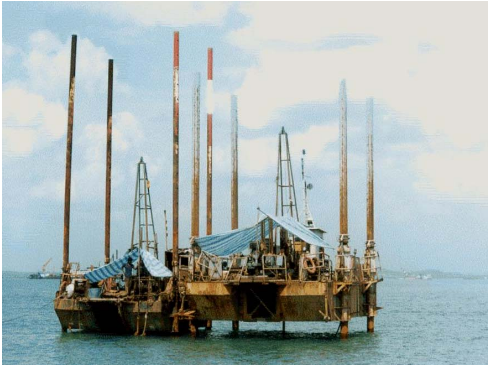
Figure 3.2 Off-shore jack-up pontoon with boring rig.
