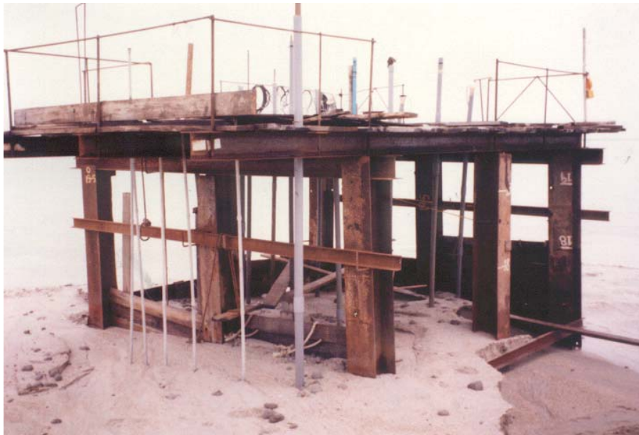
Figure 7.2 Picture of an off-shore field instrumentation platform after initial reclamation (Arulrajah et al., 2004b).
