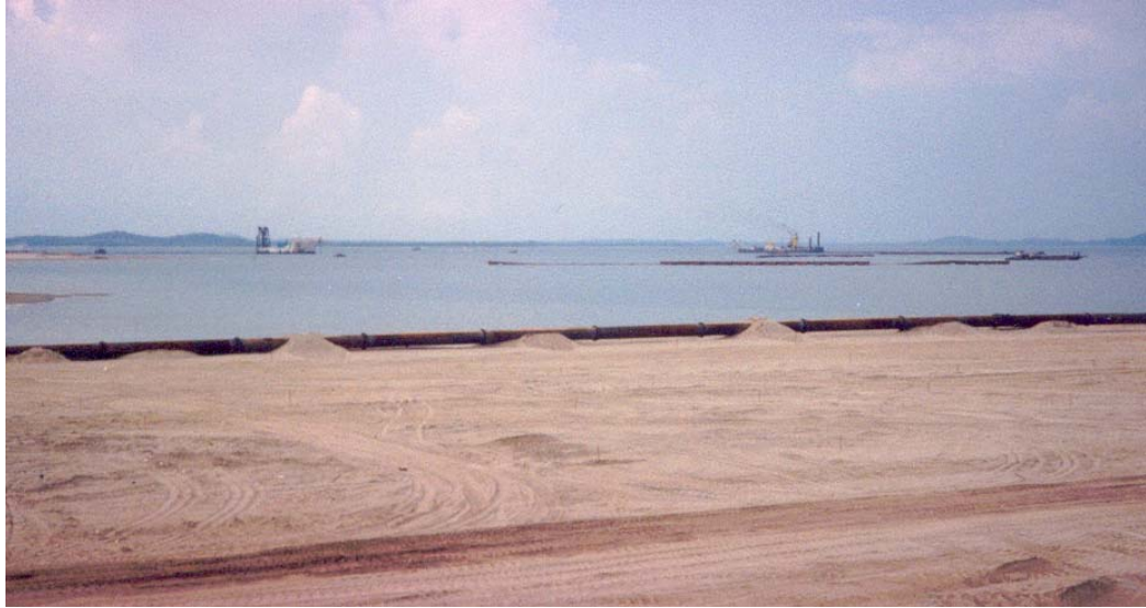
Figure 4.2 Land reclamation operations. (note cutter-suction dredgers in background).
