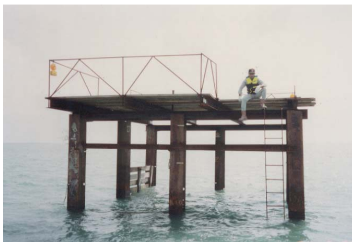
Step 3: Completion of Protection Platform
