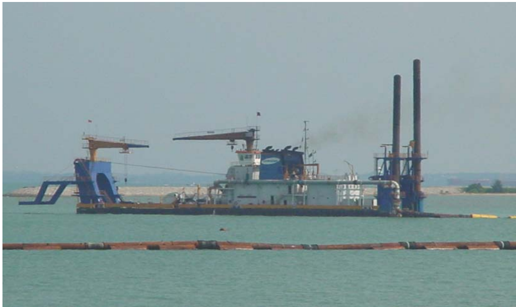
Figure 4.5 Cutter-suction dredger in operation.
