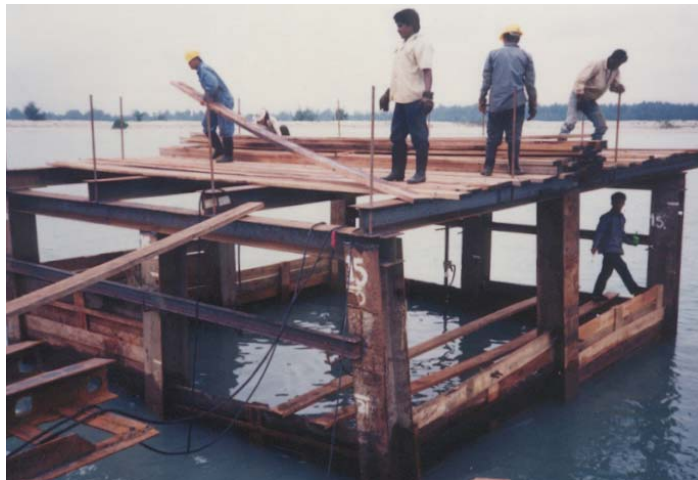
Step 2: Protection Platform Construction
