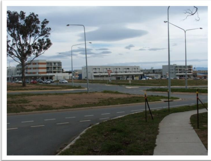
Photo 1: Gungahlin town centre medium density dwellings
