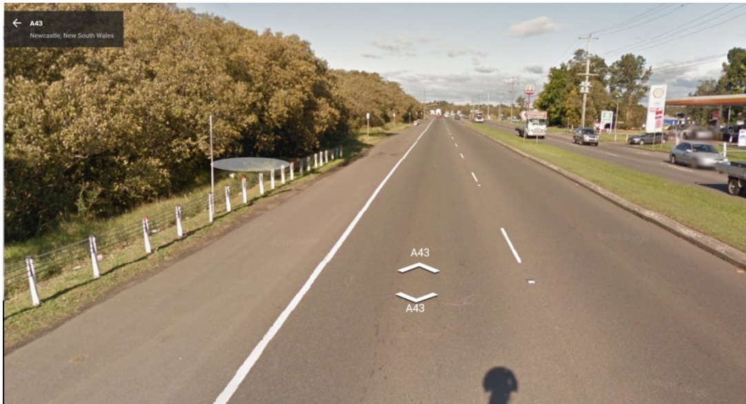
Figure 8-5 Pacific Highway, (Maitland Road) (NB)
