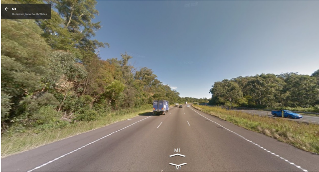
Figure 8-4 Pacific Motorway Ourimbah, (SB)
