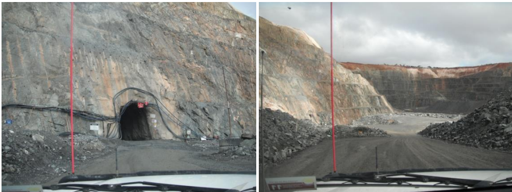
Figure 2 – Portal (mine entrance) photo. Figure 3 – Road leading to portal
