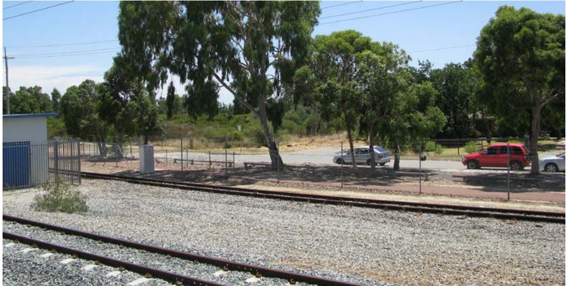
Figure 40 Deferred Urban, Kenwick Station
