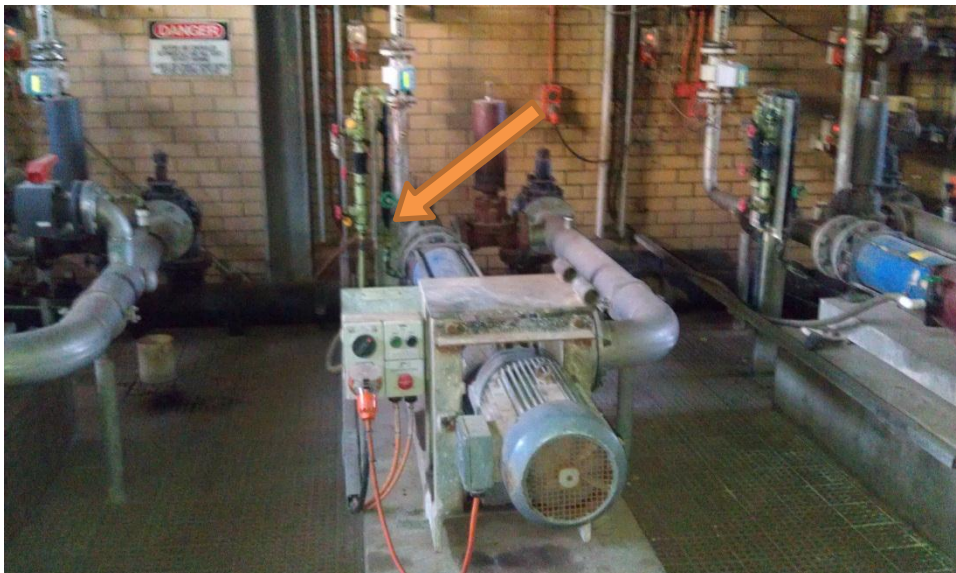
Figure 3.6: Digested sludge sampling point (centrifuge Number 2) in the dewatering section of BWWTP.
