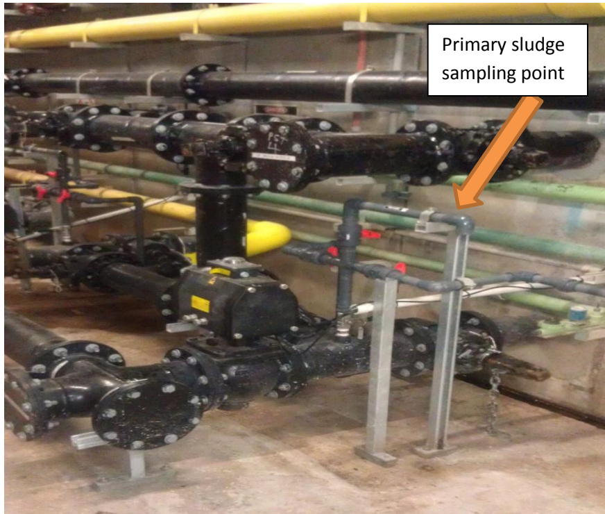
Figure 3.3: Primary sludge sampling point in the primary Gallery (BWWTP)
