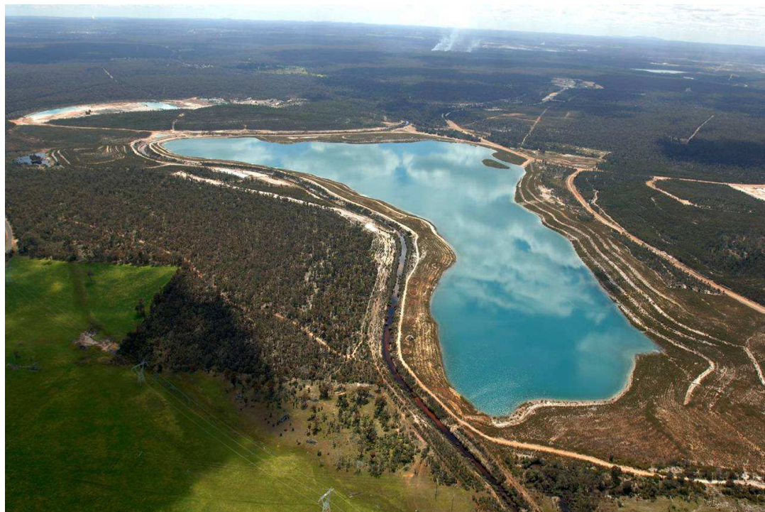
Plate 5. Lake Kepwari after filling by diversion of the Collie River. (original source unknown)
