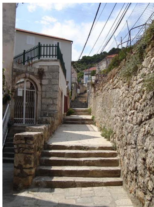
Figure 22. Retaining walls, streets and houses made out of stone. A street on the outskirts of the town of Korcula, Croatia (Glusac 2007).
