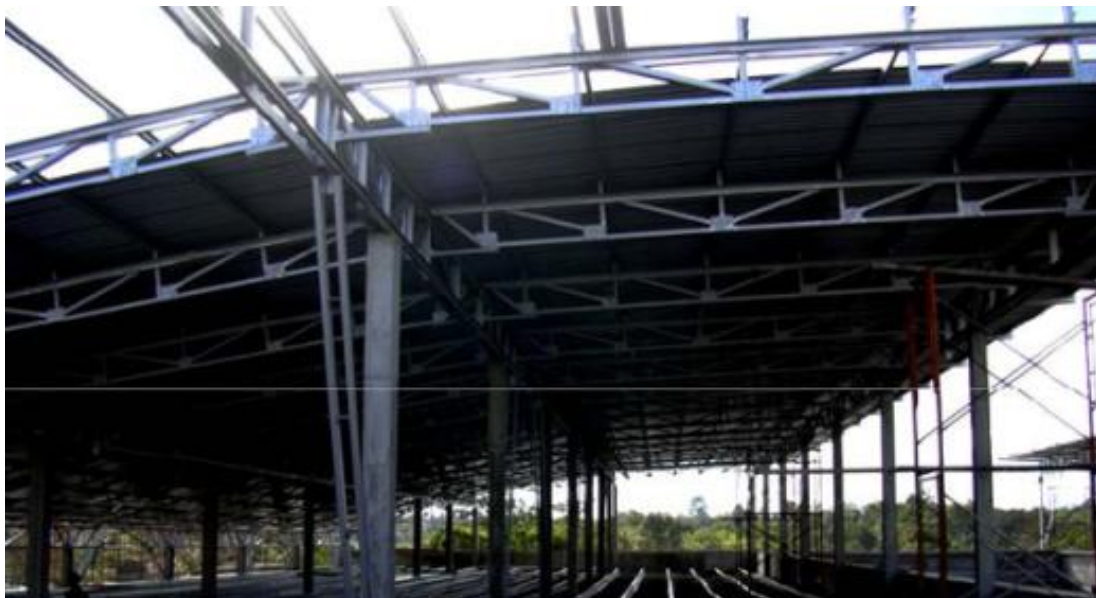
(a) Curved Roof Structure
