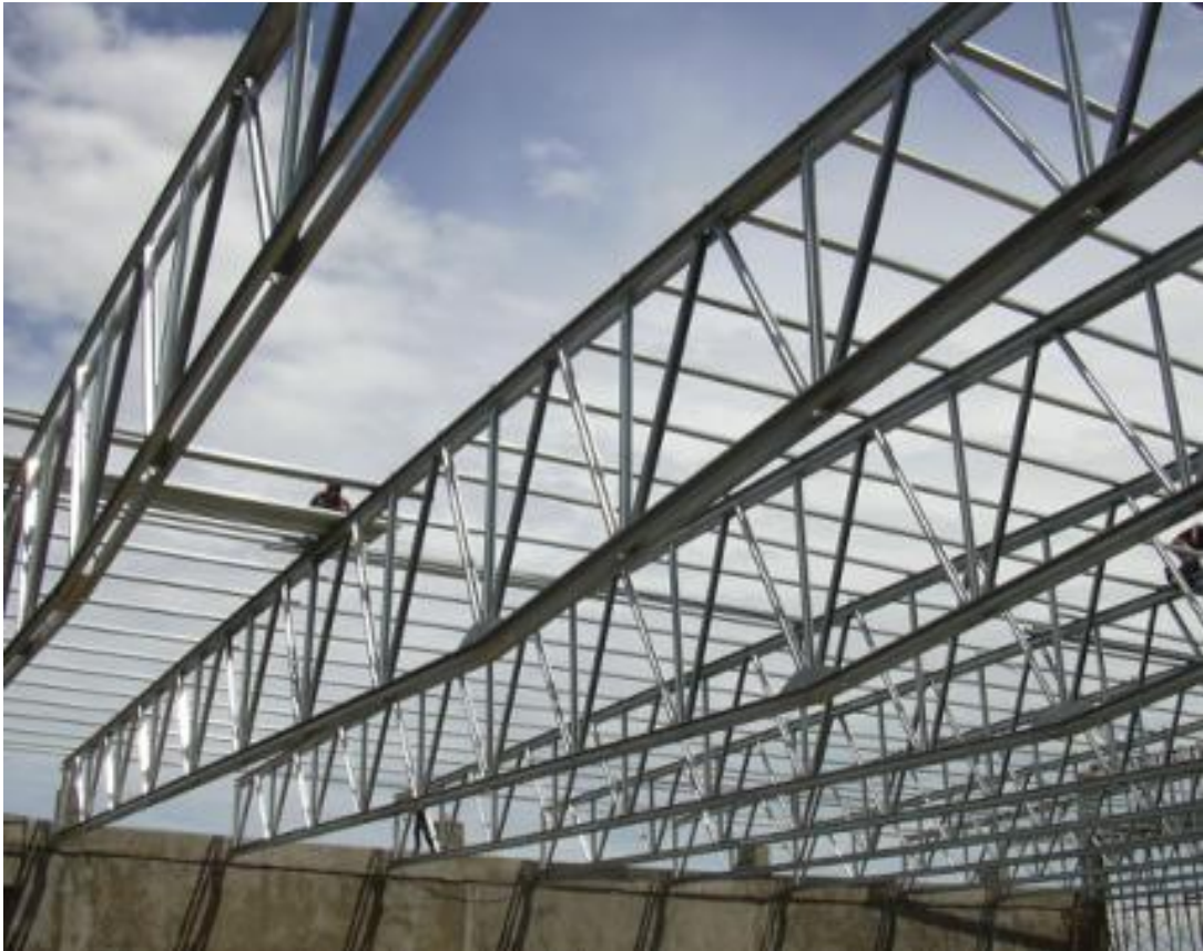
(a) Built-up Trusses
