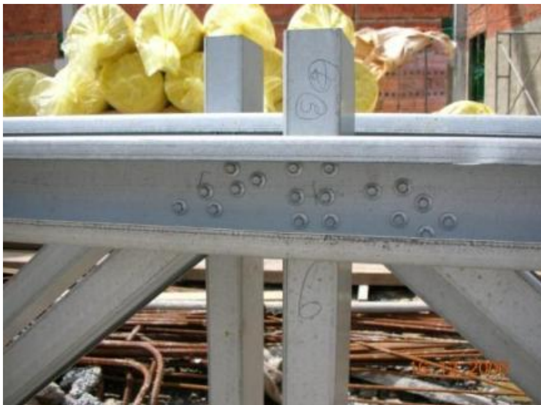
Figure 1.3: Simplified Truss Connection (Mei et. al 2009)
