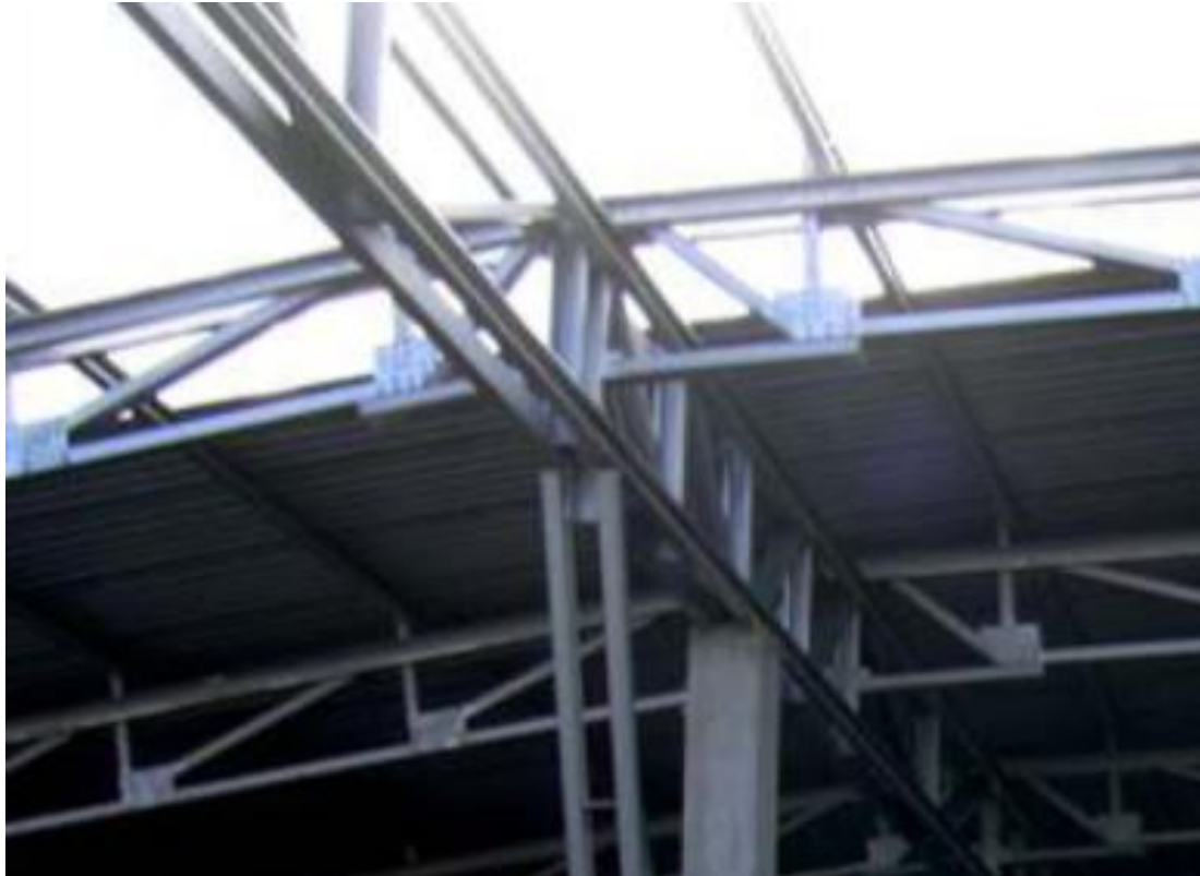
(b) Back-to-back C-channel built-up forming Curved Roof
