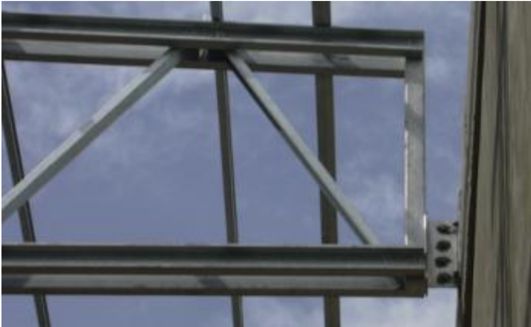
(b) Back-to-back C-channel Built-up
