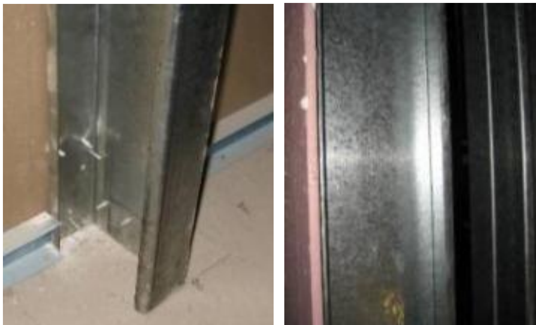
(b) Connected to Gypsum board
