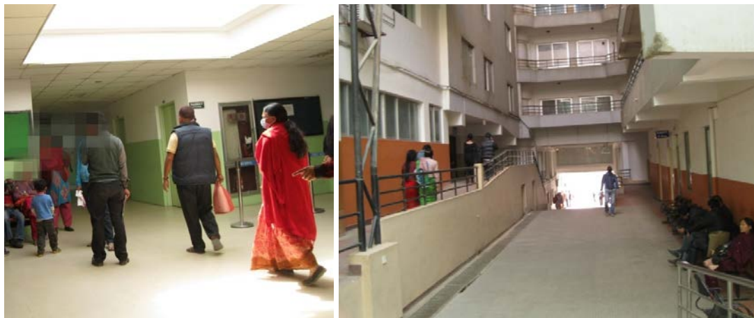
Figure 4.8: Examples of adequate and clean waiting areas (Facility 2 (left) and Facility 7 (right))
