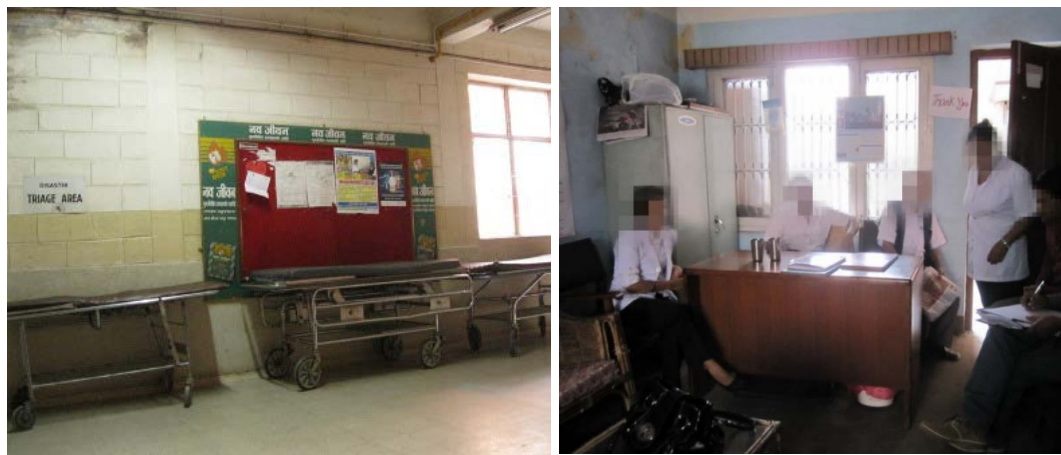
Figure 4.7: Examples of moderately maintained walls (Facility 11 (left) and Facility 12 (right))
