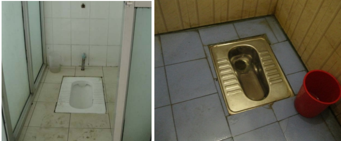
Figure 4.10: Examples of toilets maintenance (Moderately-clean toilet facility at Facility 2 (right); Very clean toilet at private Facility 7 (left))
