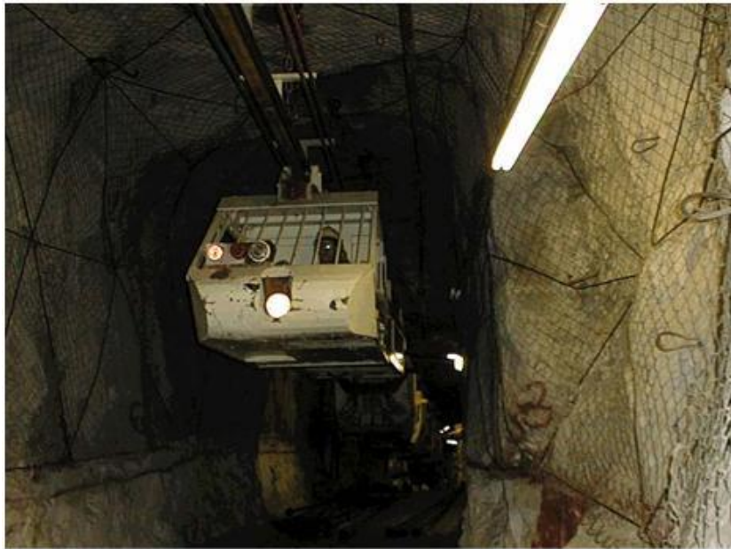
Figure 6.1: Decline support system for monorail installation (Scharf, 2007)
