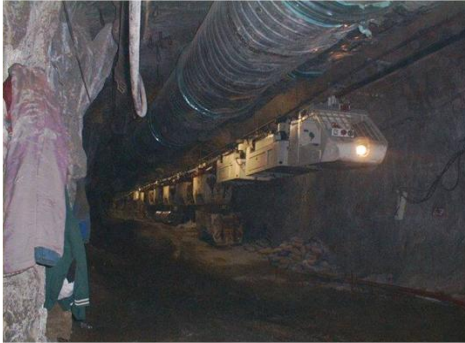
Figure 2.2: EMTS in an underground haulage (Scharf, 2007)
